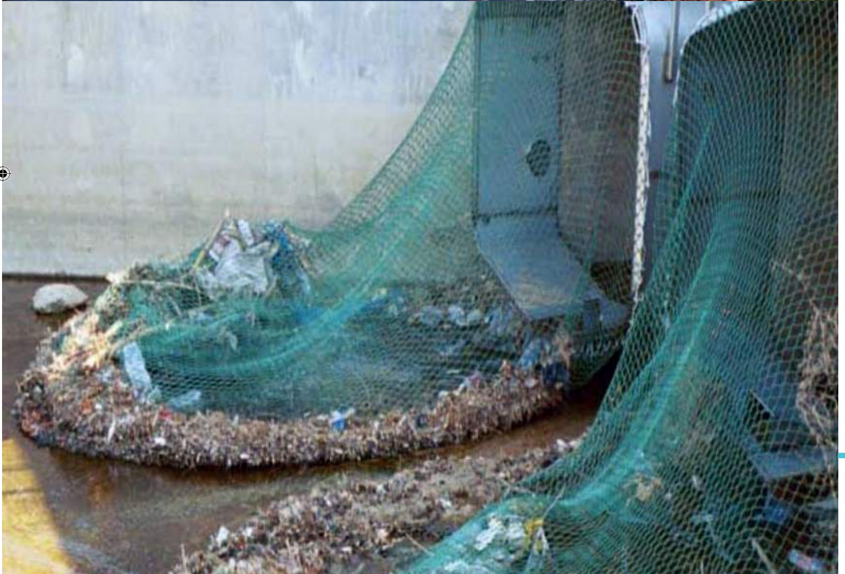
Litter traps, nets and booms are still relatively new concepts in Australia, however the USA has been leading the way in this technology for some time (Above: Watergoats, Tampa Bay / below: EPA USA netting system).
