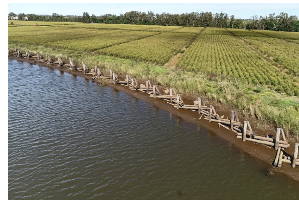
Figure 10. Log fillets, pictured here - are one of the riverbank restoration techniques specifically designed to protect the bank toe from boat wash, providing shelter for native vegetation (such as mangroves) to recover.
