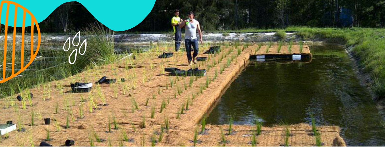
Figure 16. Floating wetlands are just one possible hybrid engineered solution to help dramatically reduce in-stream pollutants and nutrients.
