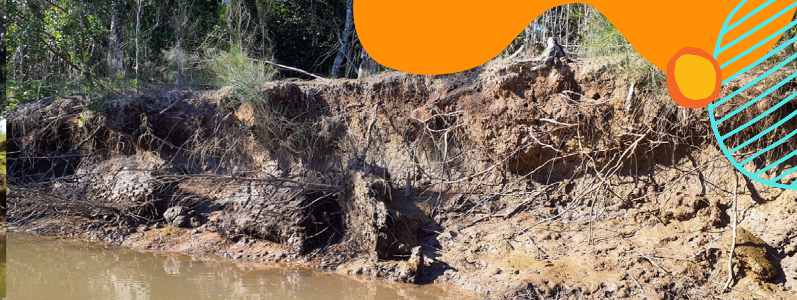
Figure 15. Heavily eroded banks showing murky, turbid, sediment-laden water below.
