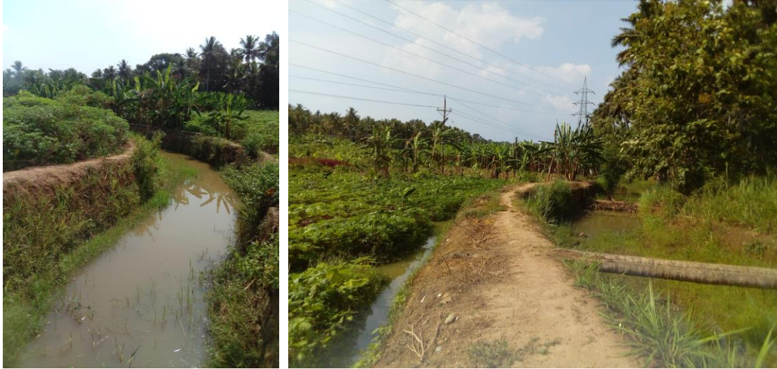
Figure 8: Main channel and irrigation channels in the upper part of the watershed
