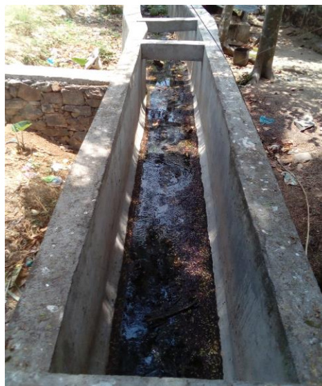
Figure 21: concrete sewage infrastructure
