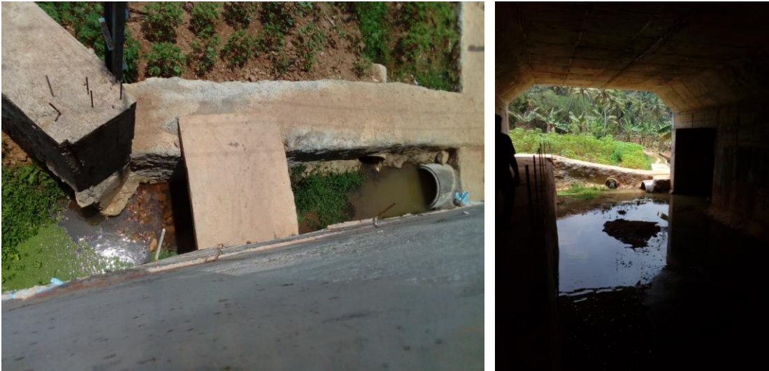
Figure 5: The river is channeled under the highway
