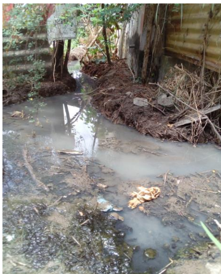
Figure 22: natural sewage channel
